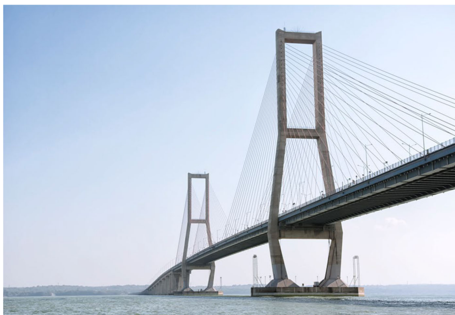
Figure 2. The Surabaya-Madura (Suramadu) National Bridge. (Source: iStock/Valens Hascaryo, 2019)
