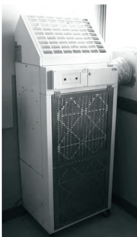
Gambar 8.8 Contoh jenis HEPA filter unit ( International Health Facility Guidelines, 2017 )
