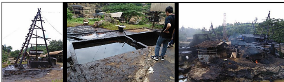
Figure 2. Crude oil exploitation facility in Wonocolo public oil fields in April 2017
