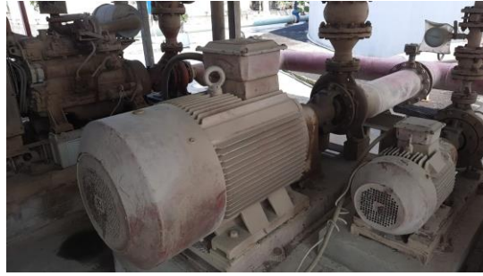
Gambar 4.9 Electric Hydrant Pump
