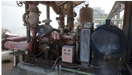
Gambar 4.11 Diesel Pump
