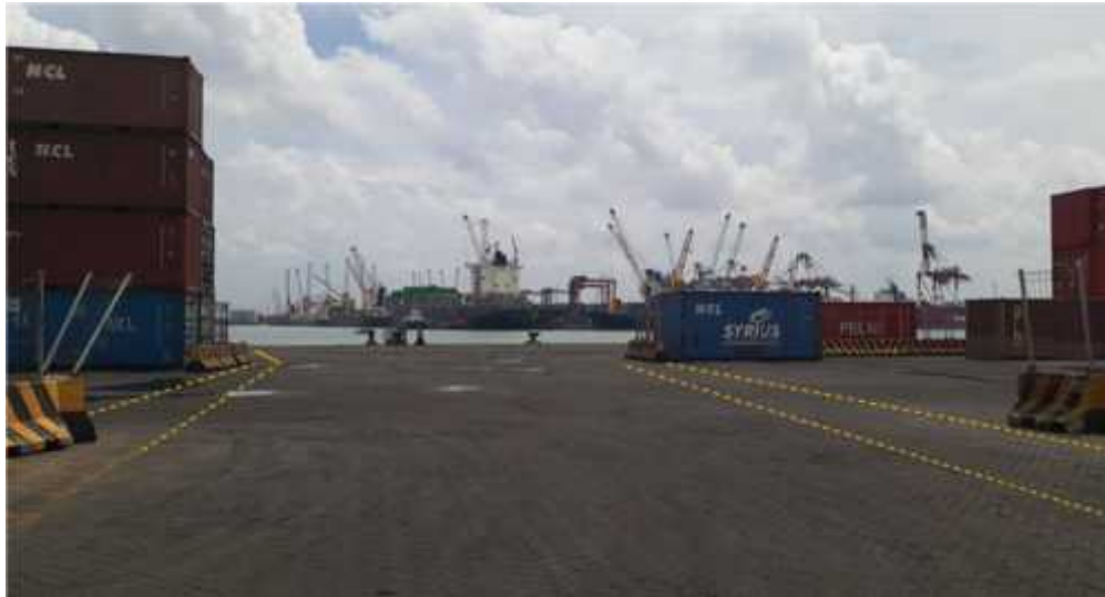
Gambar 4.9 Jalur Pedestrian Terputus Di Area Container Yard Selatan
