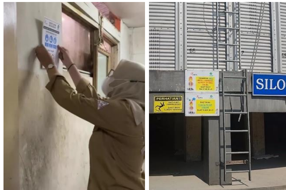
Gambar 4.4 Pemasangan Safety Sign
