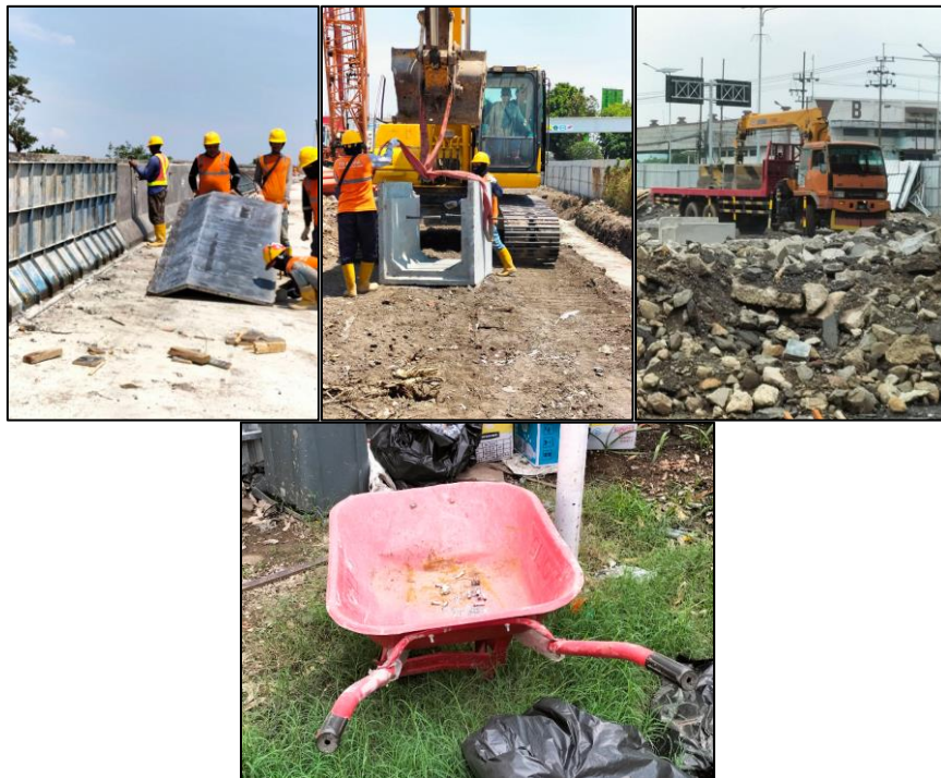
Gambar 4.10 Mobile Crane , Excavator, Bekisting Parapet, dan Gerobak Roda 1
