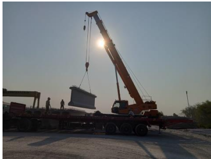
Safety patrol manual handling
