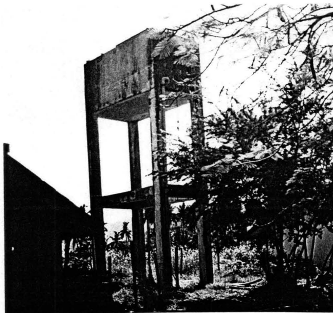
Gambar 5. Bak menara air tawar
