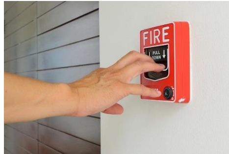
Gambar 2.6 Alarm Manual
