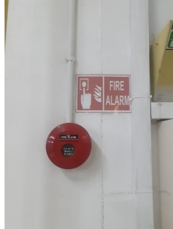
Gambar 4.17 Alarm Manual
