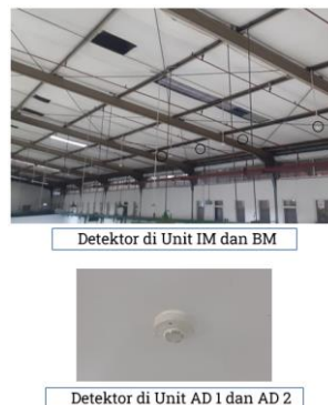
Gambar 4.16 Detektor Asap di PT. Albea Rigid Packaging Surabaya
