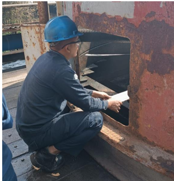
Gambar 4.2 Posisi Kerja Pekerja Maintenance Rotary
