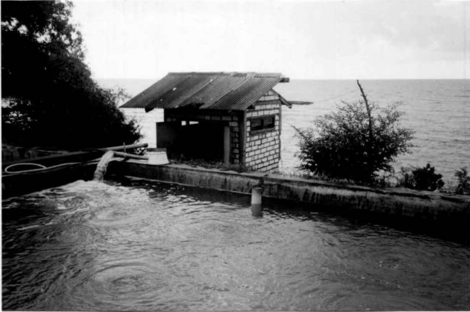
Gambar 5. Bak pengendapan dan treatment air laut di Instalasi Hatchery APS Paciran
