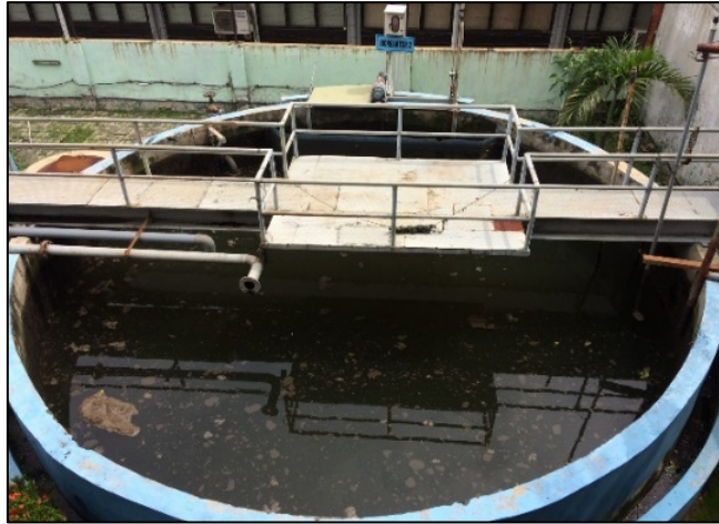
Gambar 4.10 Bak Bioreactor IPAL RSUD Dr. Soetomo
