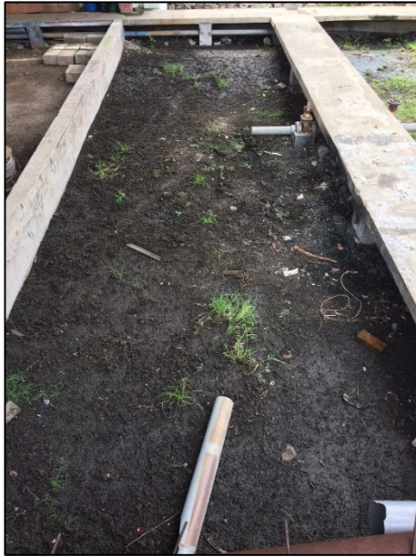
Gambar 4.11 Sludge Drying Bed IPAL RSUD Dr. Soetomo
