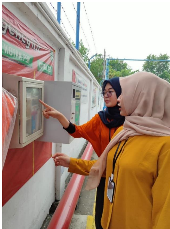
Gambar 4.48 Pengecekan Box Hydrant
