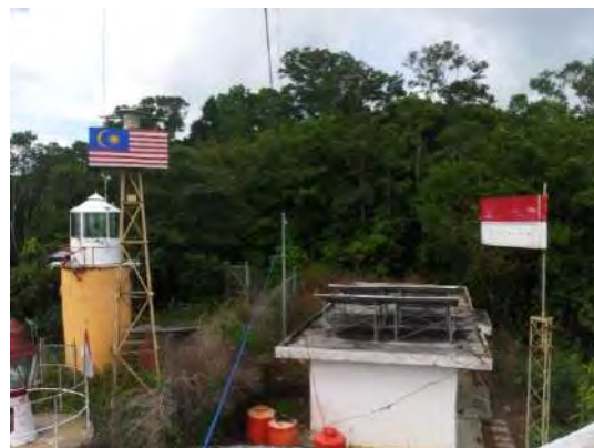
Picture 8 : Tanjung Dato' Navigation Tower
