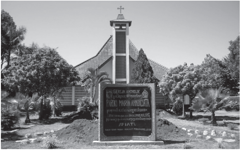
The Catholic Church of the Annunciation of Mary in Arjowilangun Village which is the subject of the study. (Photo courtesy of Hariawan Adji, O. Cam.)
