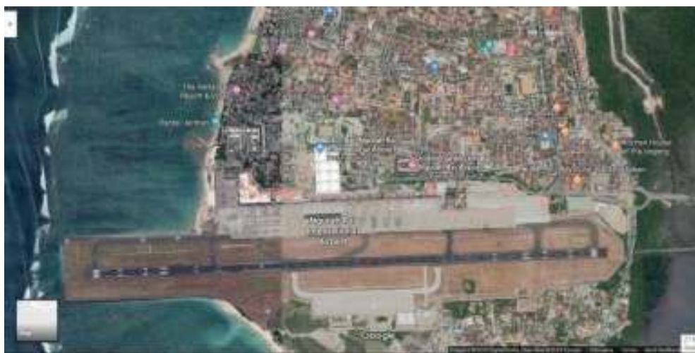
Picture 1- The office from Google Maps
